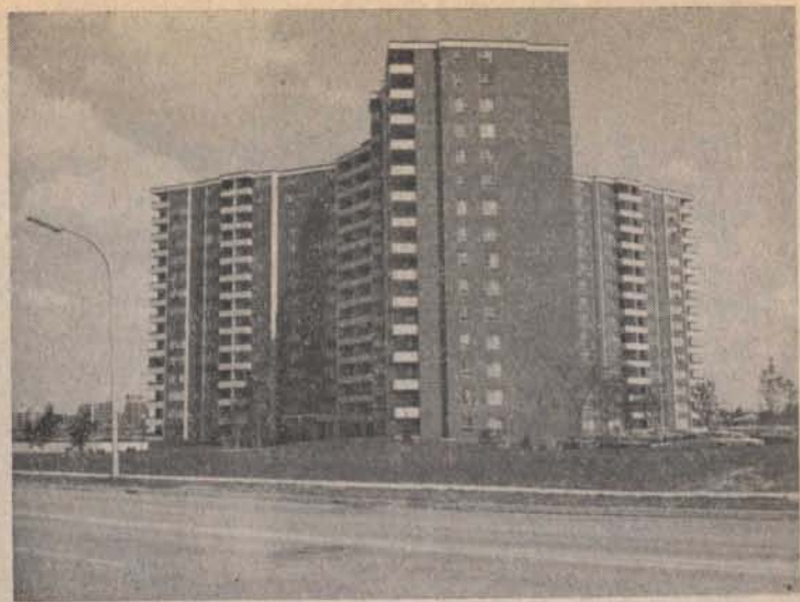
451 The West Mall, Etobicoke, Ontario, Canada
